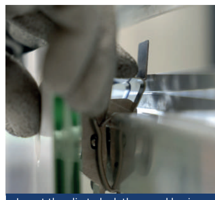
Insert the clip to lock the panel horizontally.
