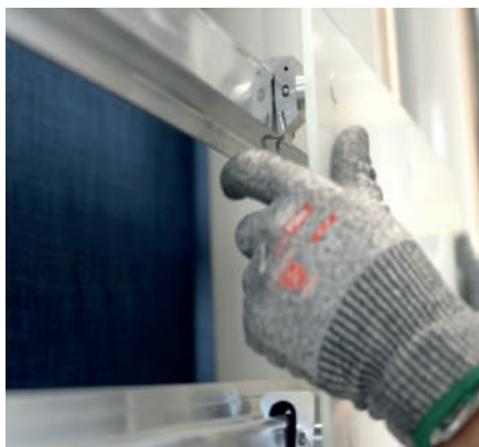
Insert the ring and screw into the countersunk hole in the panel, then tighten with the hook.
