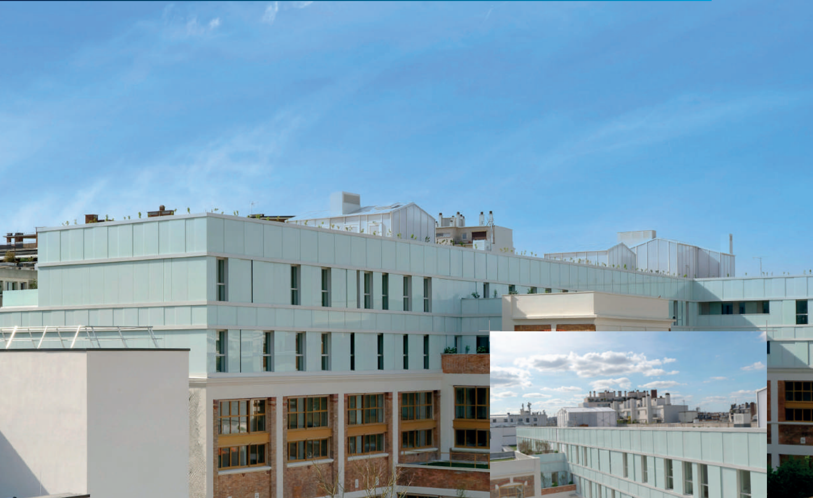
RENOVATION OF PARISTECH BUILDING - Paris
