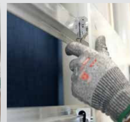
Insert the ring and the screw in the countersunk hole of the panel and screw them with the hook.
